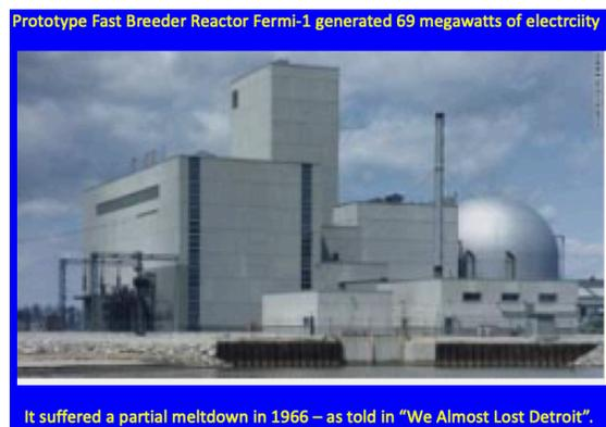
Fermi-1 reactor, 200 megawatts of heat
